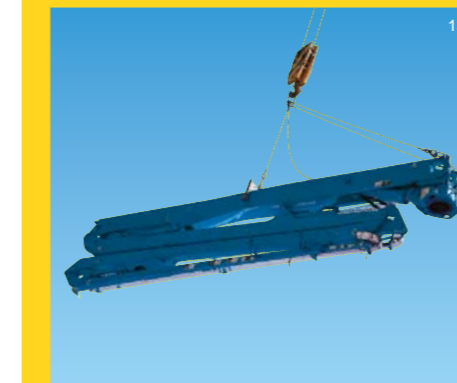
Step 3: Fly boom from truck to tower
